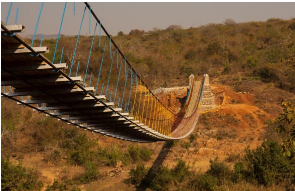
Mana Acosta and Levi Stutzman helped to build this bridge in southern Africa.
