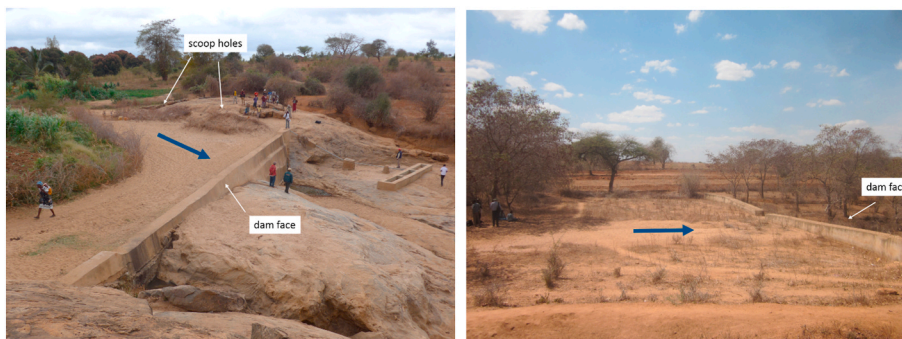
Fig. 1. Two examples of sand dams in Ukambani. Sand dam in left panel has intact dam face, functional scoop holes for water collection (surrounded by brush to exclude livestock), and evidence of green vegetation. Sand dam in right panel lacks of any evidence (such as water collection site, vegetative greening) of water accumulation, and vegetation growing on sediment surfacing suggests siltation which would limit effective storage of water. Blue arrows indicate direction of water flow. (For interpretation of the references to colour in this figure legend, the reader is referred to the Web version of this article.)
